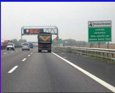
Highway data communications
